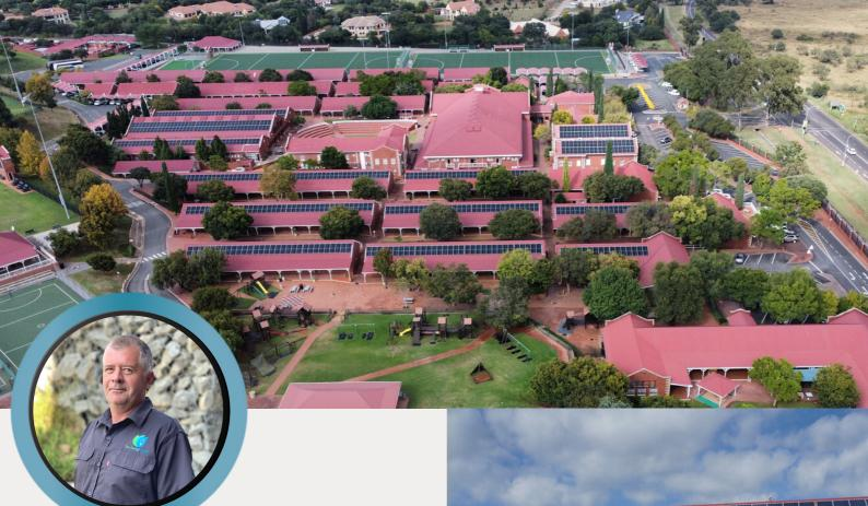
"From a time constraint point of view, we had a period of three weeks to complete an enormous amount of work namely; installation of 850 roof solar panels, installation of an 8km special cable management system, 600m of trenches that were dug by hand, 250 metres of paving that had to be lifted and replaced, installation of 3 GoodWe invertors (260kVA) and the integration of a generator.
